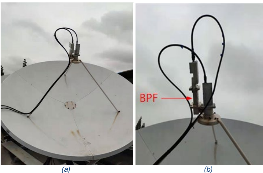
Figure 6. The AsiaSat BPF installed on one polarization of a 2.4m front-feed TVRO antenna: (a) before and (b) after the BPF installation
