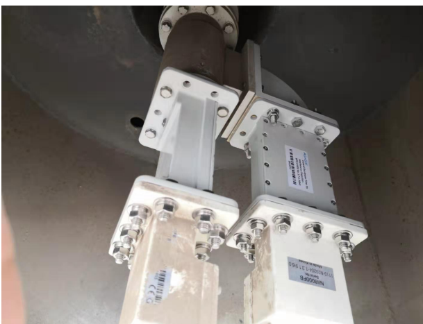
Figure 10. AsiaSat BPFs installed on two different antenna feeds. Both the V and H-polarization paths are installed with AsiaSat BPFs
