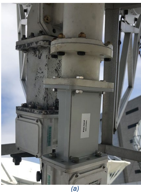
Figure 4. AsiaSat BPF tested in Tai Po, Hong Kong, in conjunction with a 3.7m TVRO antenna. (a) The filter connected in between antenna OMT output and the LNB input, and (b) The tested TV carrier MER degradation over the frequencies and channels
