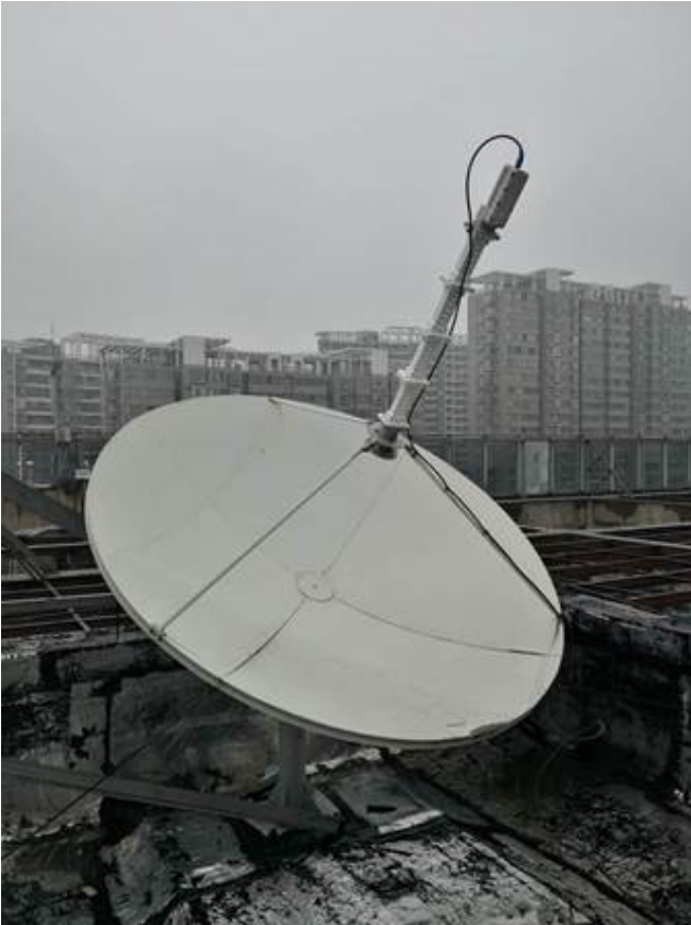
Figure 3. An inefficient ad-hoc filter(s) solution against 5G interference (photo provided by our customer)
